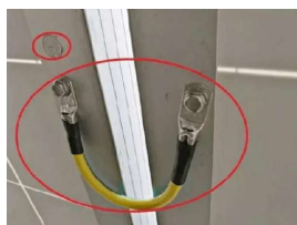
Connect the ground wire between the solar panels
